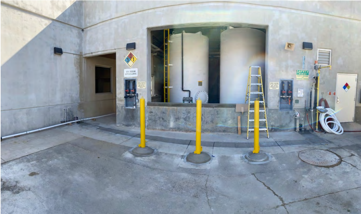
Figure 1: Lower Chemical Room Tanks 1 and 2; Replaced bollards
